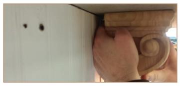
18. While holding the Mounting Base in place, remove the corbel. The top flange of the Mounting Base should be about 1/16" below the countertop surface. When installed, that space
