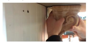
17. Position the corbel where it is desired, and with your hand between the corbel and the Mounting Base, push it against the mounting surface, making sure that the top of the corbel is touching the bottom of the countertop.
