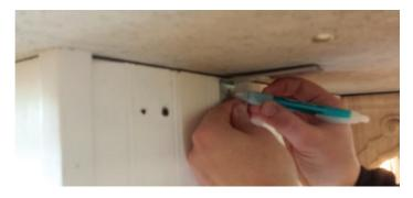
Base should be straight up and down and be level across the top flange as well as down the top flange.
