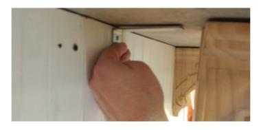
21. Attach your first Mounting Base to the substructure using the screwdriver or power drill with screwdriving bit and #8 x 2.5" wood screws. Make sure that when you fasten the Mounting Base that you check for level in all directions. The Mounting
