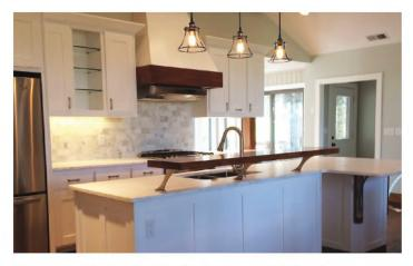
We suggest that you space the Foremont style bracket no greater than 30" apart on a standard application. With your fastening the holes prefabricated into your sub counter you can attach your first bracket. Make sure that when you fasten the bracket that you check for level in all directions. The bracket should be straight up and down and be level across the top flange as well as down the top flange. This will give the bet possible support result to your countertop.
