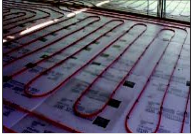
Radiant floor heating systems can save up to 50% of the heating expenses in a bath.
