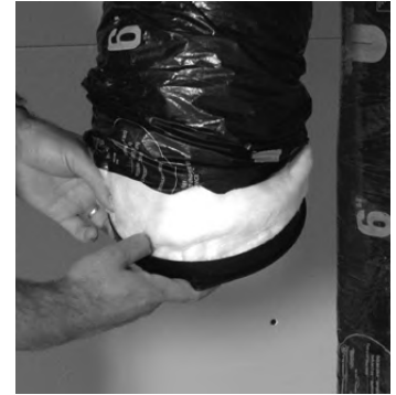
figure 7.2 Insert insulation inside the collar.
