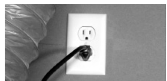
figure 9.2 It is recommended that the HRV have a dedicated receptacle with 115v. It is not recommended to connect unit with an extension cord. If no receptacle is available please call an electrical contractor and have one installed. Insure polarized is correct
