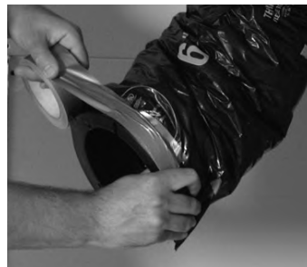
figure 7.3 Finish by taping the duct on the collar.
