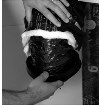
figure 7.1 Insert vinyl duct over the hooks and seal with a Tie wrap.
