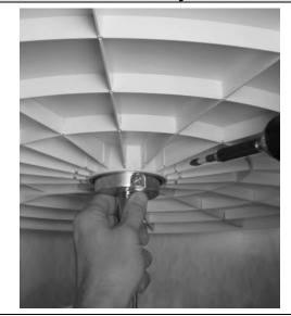
Holding onto the lower pole, twist the upper pole counter-clockwise to release. Extend pole upwards until it rests firmly against the Top Mounting Support and tighten by turning the upper pole clockwise.
