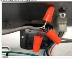
B Put the wire nuts inside the connection box base, then snap the connection box lid on its base, ensuring the ADA cable runs through the open notches.
