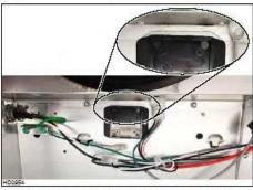
remote ADA switch outside the hood (step 1). IMPORTANT: Leave a cable length of at least 12" that protrudes from the wall (at the same location of the 120 V house wiring). Run one end of the remaining section of the ADA cable though the range hood wire clamp, along with the power cable, giving enough length to make the connections inside the box. Tighten the wire clamp, then strip the end of the 3 wires from both ADA cable ends.
